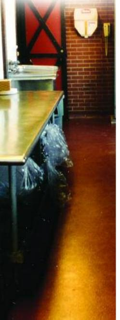
FloroCrete is a thick, heavy-duty system that is designed for the most strenuous uses and activity. It is specially formulated for use in industrial-plants and kitchens where thermal shock is an issue. FloroCrete can be maintained by using a stiff mechanical brush and/or hot pressure washer or steam cleaner.
